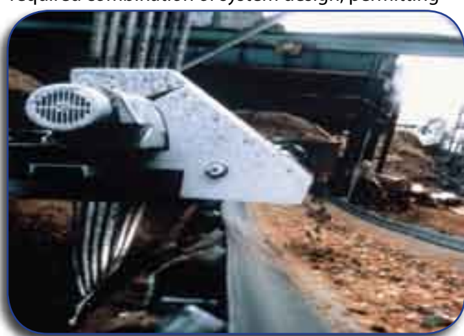
Conveyor belt to introduce wood and TDF into boiler system Photo courtesy of Terry Gray, TAG
